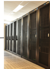
Remote data center
