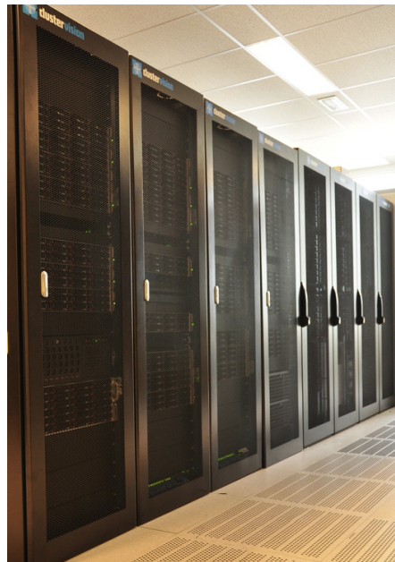
In the server room/data center
