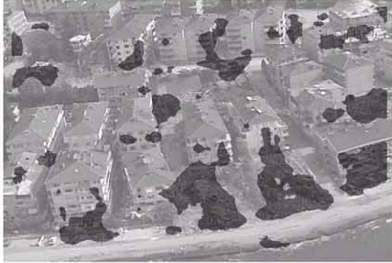
Fig. 1. Building damage distribution obtained by the automated detection
