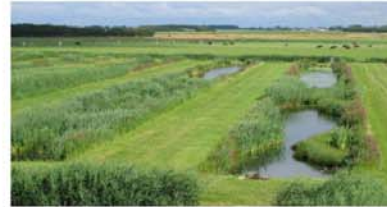
The Eversteekooog constructed wetland (Island of Texel, The Netherlands) receiving well treated waste water: massive growth of Daphnia in the 4.400 m 3 pond
